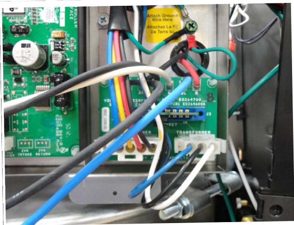
Power Distribution Board Conversion from 240 VAC to 120 VAC
