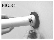
This lens assembly should glue directly on 1 1/2" PVC pipe. DO NOT GLUE A REDUCER BUSHING INTO THE LNS-A! If you want to reduce to 1" PVC pipe, do so with a reducer after a few inches of 1 1/2" PVC pipe. This is to allow room for the lens assembly to seat into the body of the lens housing.
