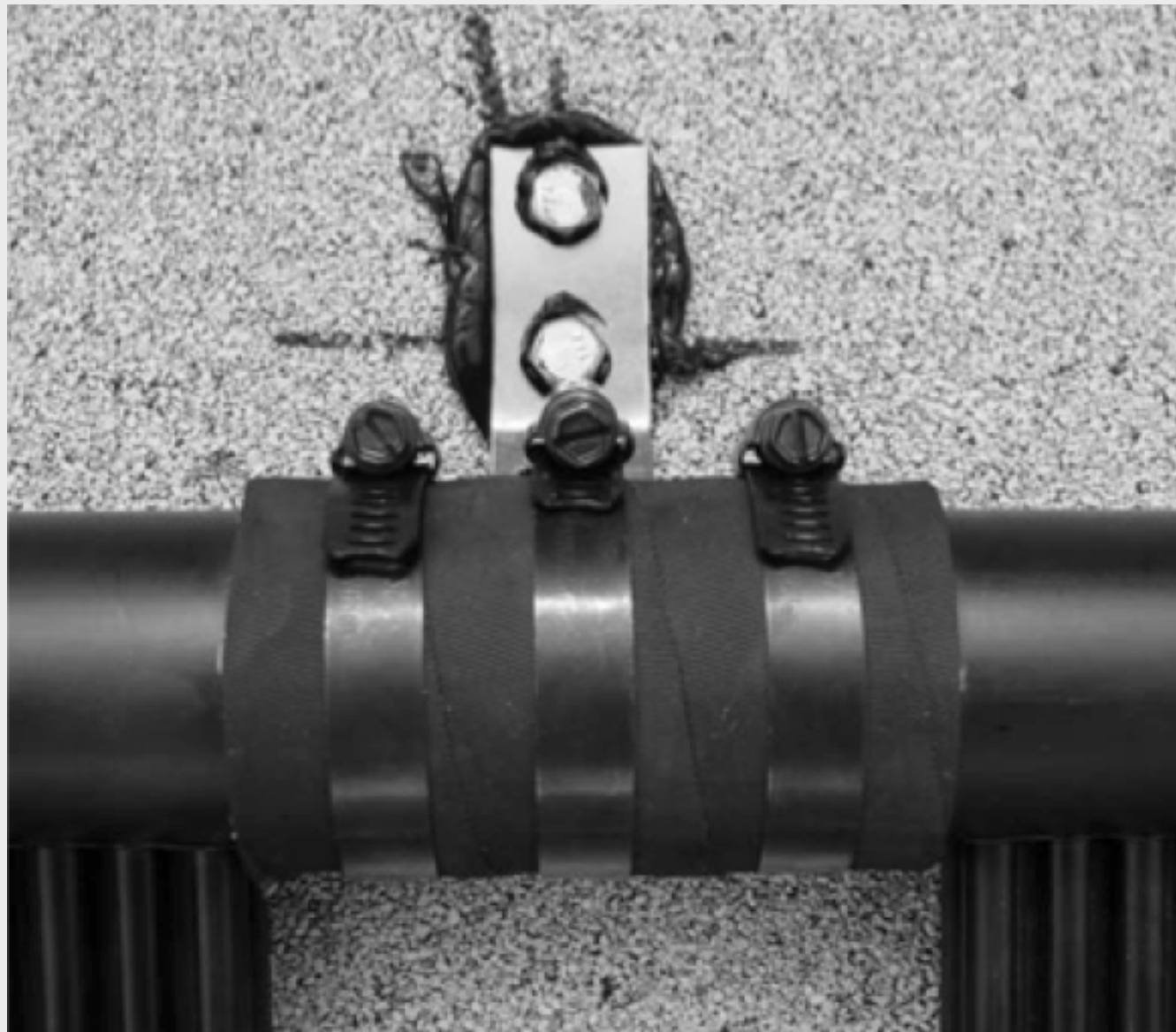
FIGURE 5 Installed Outlet Header Bracket with Hose
