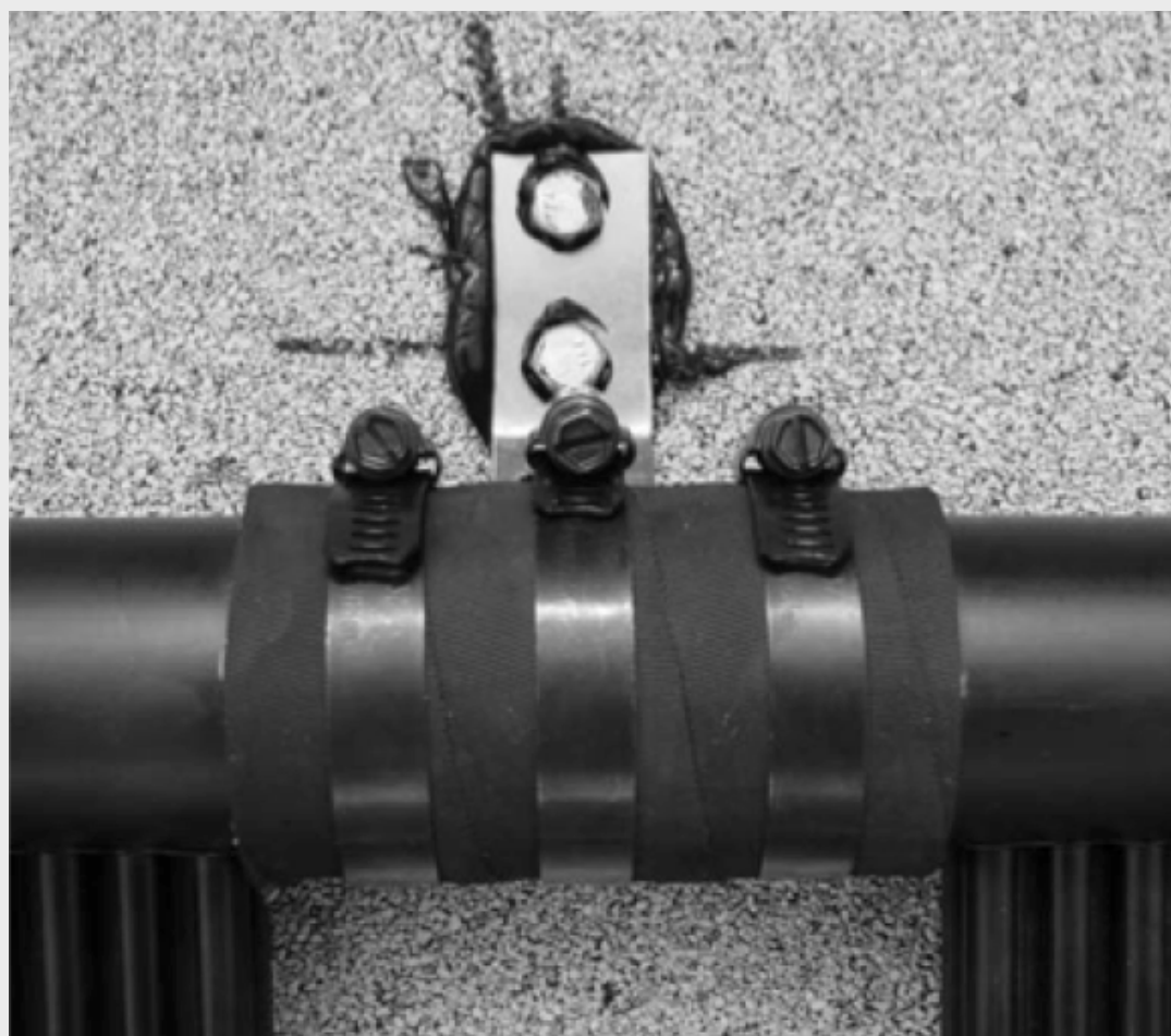
FIGURE 5 Installed Outlet Header Bracket with Hose
