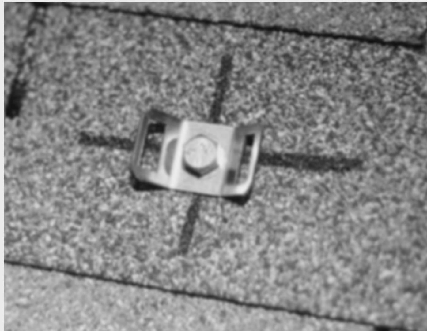
FIGURE 6 Hold-Down Strap Bracket
