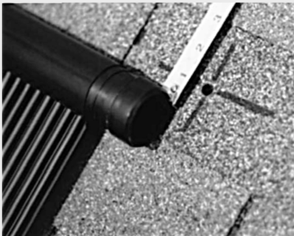
FIGURE 3 Outlet Header Bracket Location
