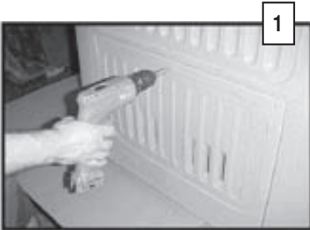
1 Remove and save access panel screws. Use caution when reinstalling the screws. Do not overtighten.
