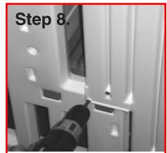
Fasten using eight (8) #10 x 1-1/4" screws at the pre-marked locations on both sides of hinge mounting post.
