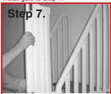
Spread open the flange of the hinge mounting post and slide down over the right gate adapter post (*installed in step #2*) until it comes into contact with side panel.
