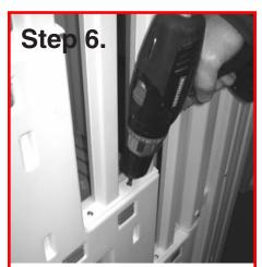
Fasten the bottom of the pickets to the step unit at the pre-marked locations using twelve (12) #10 x 3/4" screws.
