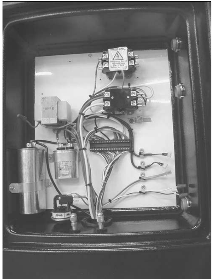
Figure 13. AE-Ti Control Panel, Interior View
