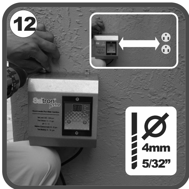
Failure to mount the power supply vertically will void warranty
