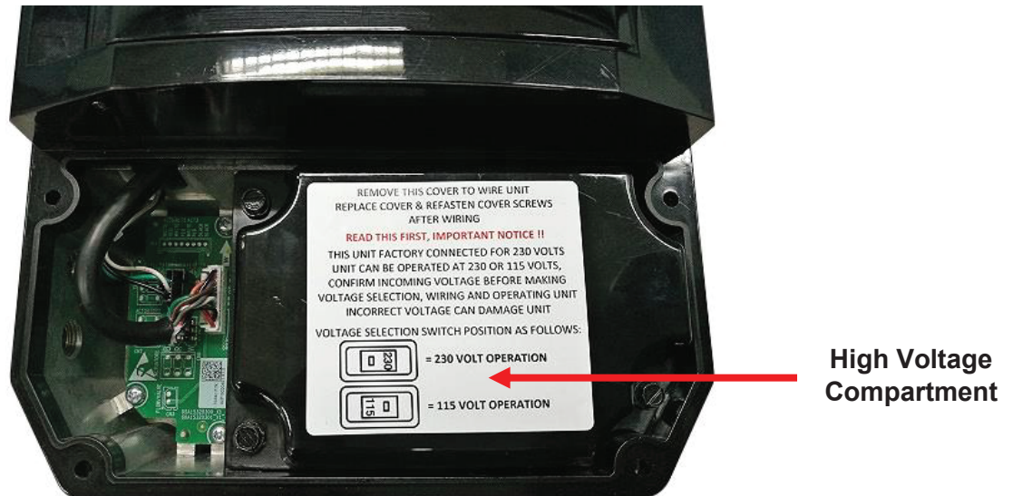
Figure 1 – High Voltage Compartment
