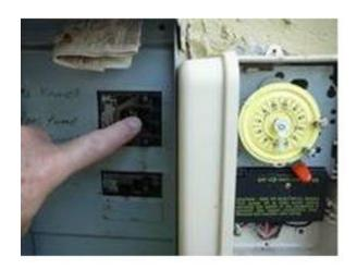
Step 2 Loosen the four screws from the terminal cover and remove the terminal cover plate.
