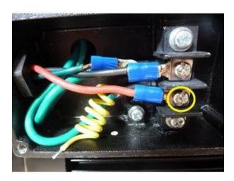
Step 6 Connect the green (ground) line to the yellow wire using a wiring nut.
