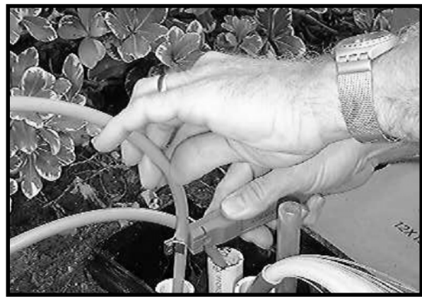
2. Strip jackets from 0 to 2 in. above the base.
