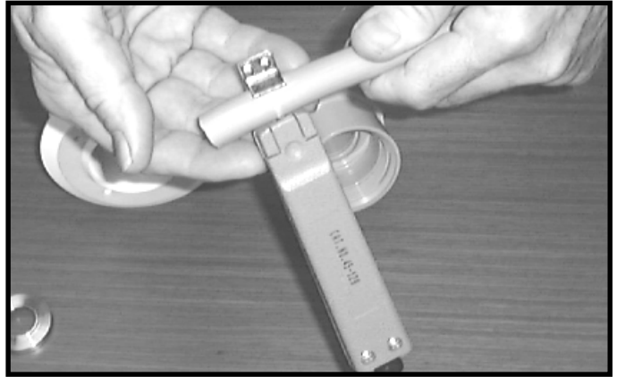
1. Remove 1 in. of the jacket with the stripper.
