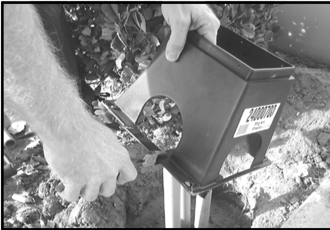
2. Cut sub-base flanges as needed.
