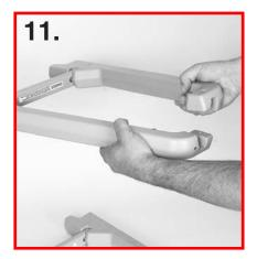
Connect the two handrail returns to the handrail connectors.
