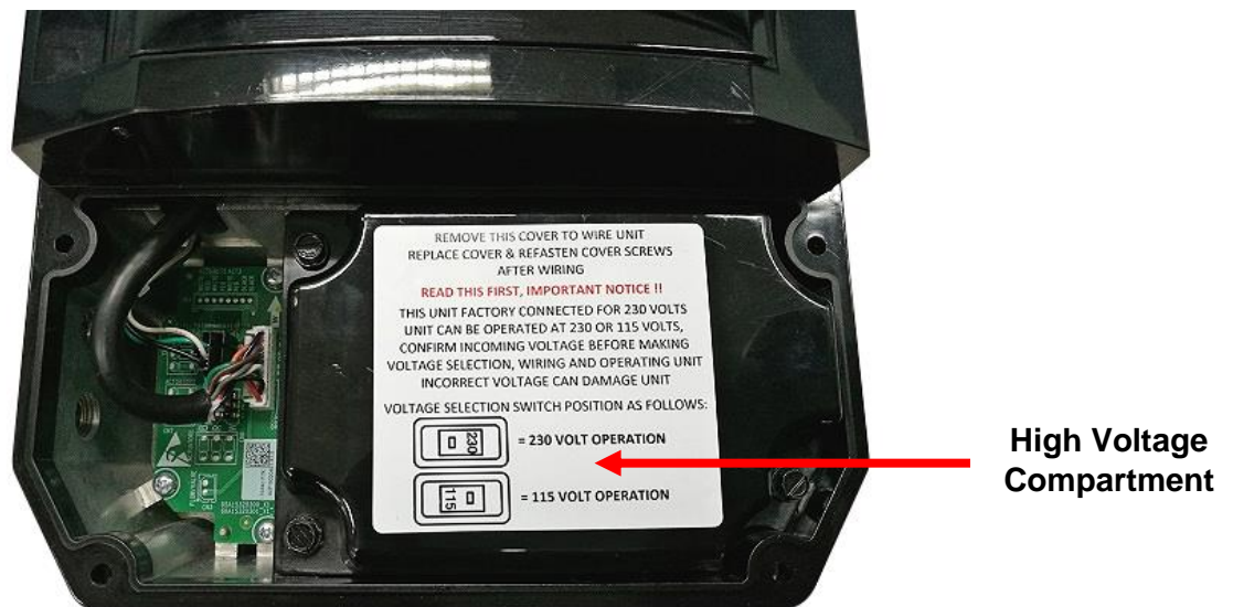
Figure 1 – High Voltage Compartment
